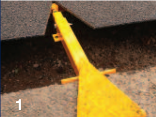
Move the roadplate into position.
