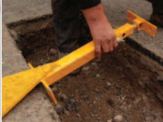
Place PlateLOK across the trench or excavation.
