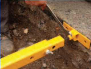
Ensure the bolt is tightly fastened.
