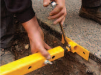
Using a 24mm spanner, gradually tighten the adjuster bolt.
