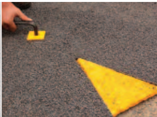
Tighten using 16AF hex-key.
