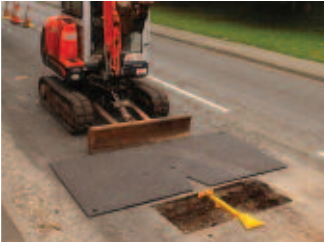
Move the roadplate into position.
