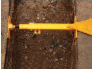
The PlateLOK is now ready to receive the roadplate.
