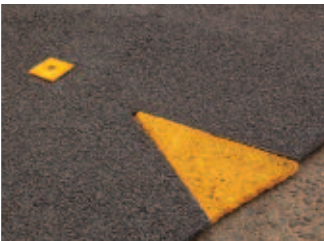
The completed installation.
