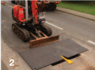
Move the roadplate into position.
